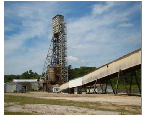
*Mine elevator and wooden conveyor gallery system. The two models are: 500M at 20 HP and 480 fpm with 31.5" face width and 630H at 60 HP and 600 fpm with 37.4" face width.*
